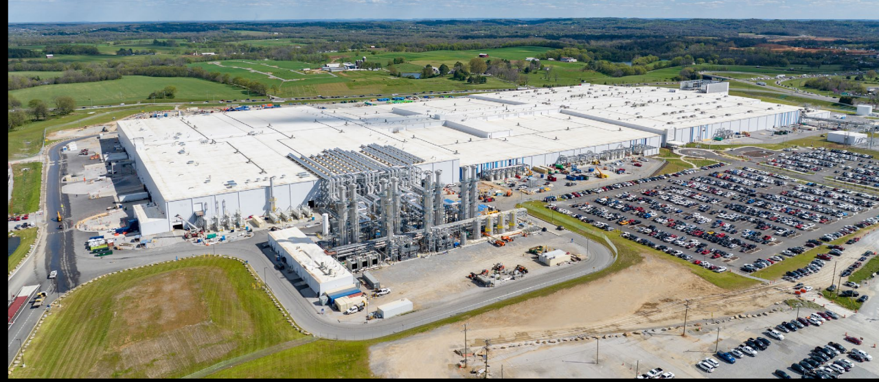
Ultium Cells, EV Battery Manufacturing Plant, Phase 2, Spring Hill, TN 2,800,000 sf | 156 acres | 30 GWH Annual Capacity | $2.3B Investment
