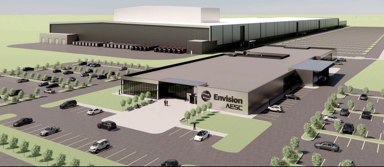
Envision AESC, EV Battery Manufacturing Facility, Bowling Green, KY 1,500,000 sf | 500 acres | 30 GWH Annual Capacity | $2B Investment
