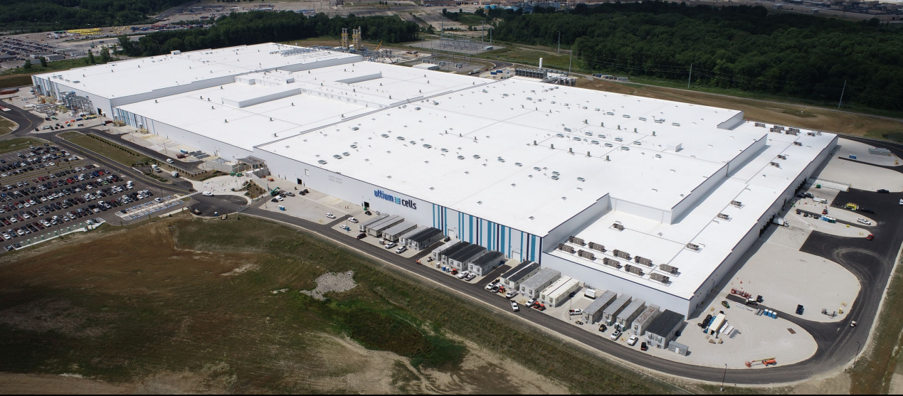
Ultium Cells, EV Battery Manufacturing Plant, Phase 1, Warren, OH 2,800,000 sf | 156 acres | 30 GWH Annual Capacity | $2.3B Investment
