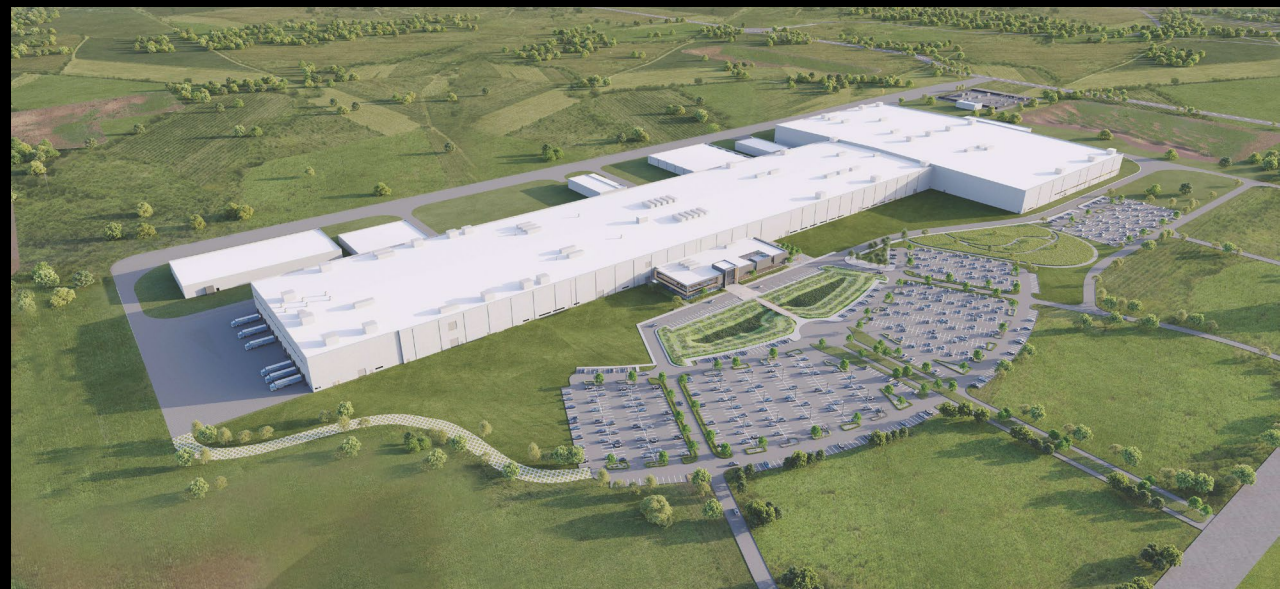
Project Amplify, EV Battery Manufacturing Plant (LFP) | Marshall Co. Mississippi 2,000,000 sf | 21 GWh Phase 1 Annual Capacity | Commercial Vehicles
