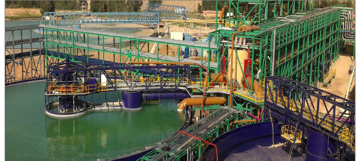
Traditional Pyromet Plant
